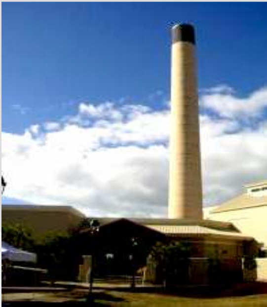
The old Waipahu Sugar Mill – a local landmark – sits in back of the Leeward YMCA's six-lane heated pool.
